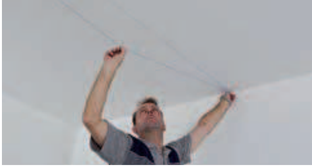
Mark out the ceiling module from the centre of the room, for example using a chalk line. Ensure the margins at the sides of the room are identical.
