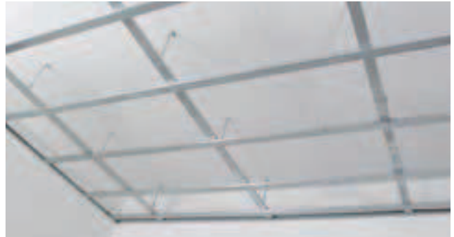
Finished ceiling grid.
