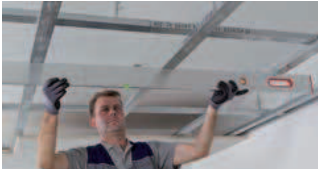
Align the CD-profiles using a spirit level or laser level.
