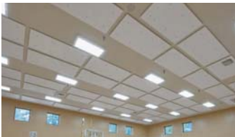
Camo Application (CA) Direct Screw to Furring Channel or Drywall Grid (Visible screws)
