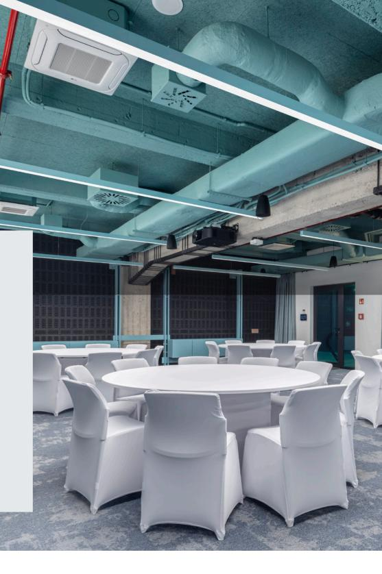
The Knauf Ceiling Solutions HERADESIGN<sup>®</sup> wood wool ceiling tiles proved to be the ideal choice, offering a perfect balance of aesthetic and performance. Specified here in a palette of greys and natural tones, these panels perfectly blend with the building's brutalist look and provide much needed acoustic support to help open spaces perform as well as they look.
